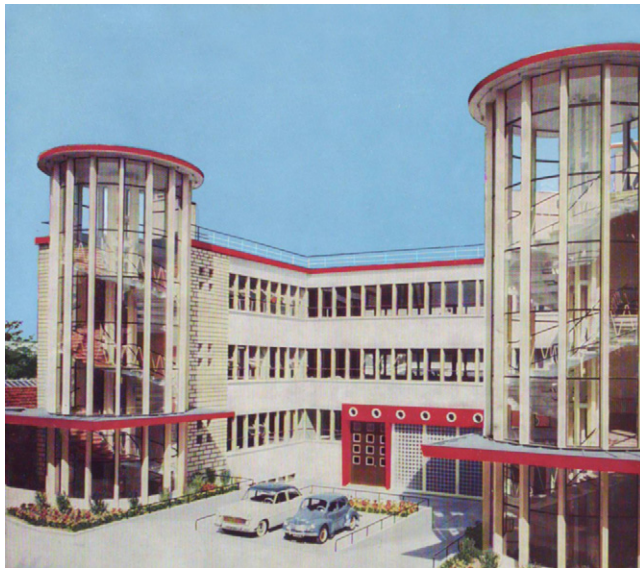
FIGURE 10 The Cameca plant in Courbevoie, as it is on the picture, with two towers, was built in 1956. The photograph dates from 1960.
